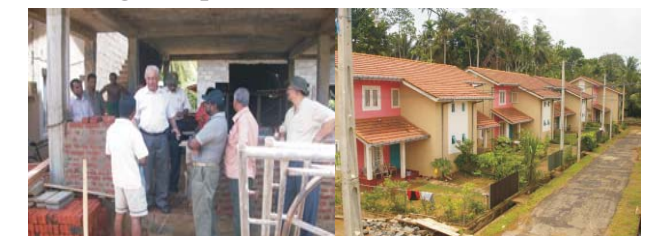
New Community Centre Aththiligoda Housing Project Under Construction
